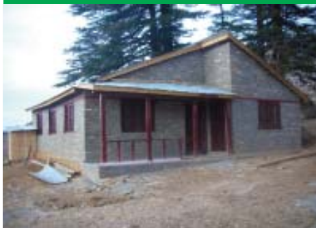
Health post building of tamti Jumla
