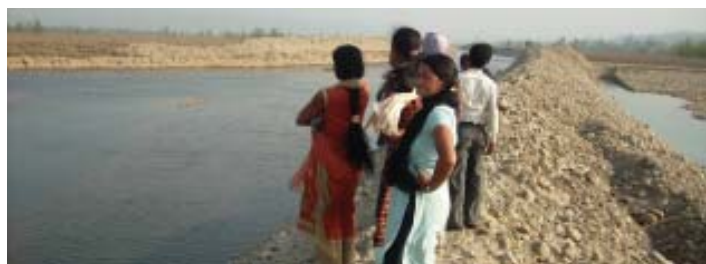
Embankment built by Affected People’s Network on Kamala River in Sindhuli
