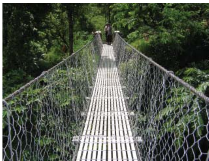
A suspended bridge in Nuwakot
